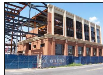
Construction underway – wall sections in place
