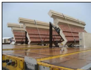
Modular pre-cast concrete wall sections clad with Robinson Brick Thinbrick
